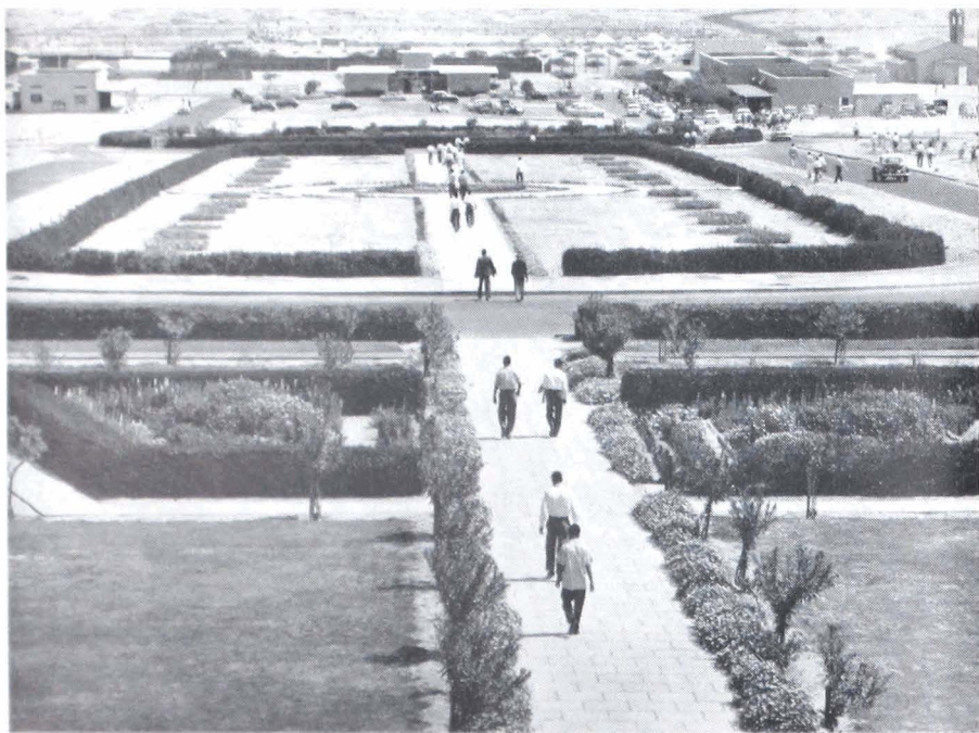
VIEW OF THE KUWAIT OIL COMPANY'S MAIN OFFICE LOOKING TOWARDS THE DISPLAY CENTRE, AHMADI MARCH 58
